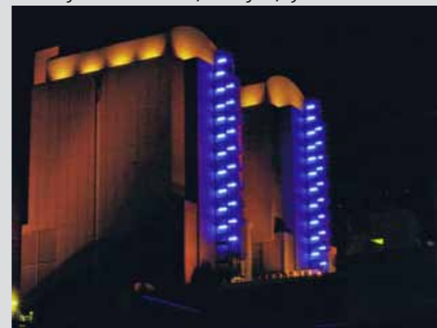
Westhafen Powerstation, Frankfurt, Tyskland.
